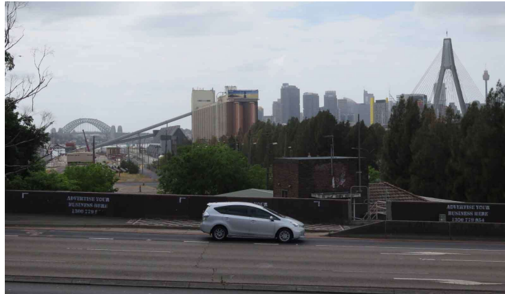
Figure 20 – View looking east from the Victoria Road overpass near Lilyfield Road showing the subject Glebe Island Grain Silos, Anzac Bridge and Sydney Harbour Bridge. Victoria Road is visible in the foreground (Source: NBR SARCHITECTURE, October 2017)
