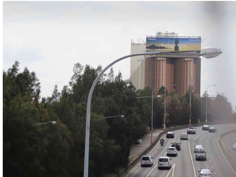
Figure 16 – View east looking from the overpass over the Western Distributor and approach to the Anzac Bridge showing the west elevation of the silos painted and advertising mounted on the upper level (Source: NBRARCHITECTURE, October 2017)
