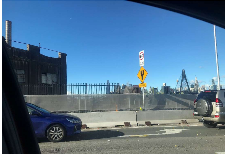
Figure 21 – View looking east from the Victoria Road overpass road deck, showing the relationship between the Anzac bridge, the Silos and the White Bay Power Station (the structure to the very left of the image). (Source: NBR SARCHITECTURE, June 2021)
