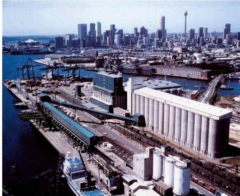
Figure 11 – Glebe Island Silos, pre-2000. This view shows the north-eastern elevation of the subject bank of silos at centre right. Note the structure perched on top of the silos and the northern tower. (Source: Flickr, https://www.flickr.com/photos/59203598@N00/14624518444 )
