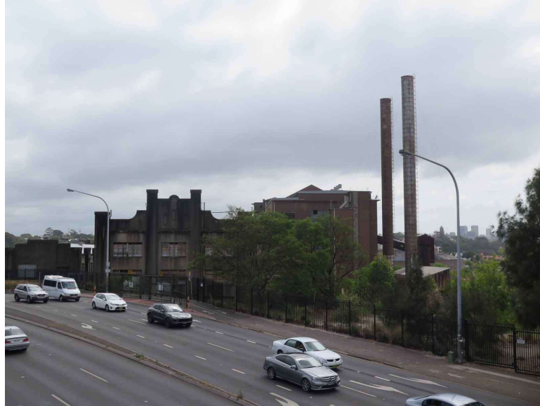
Figure 14 – View looking northeast from the Victoria Road overpass near Lilyfield Road to White Bay Power Station, a heritage item of State significance, located north of the Glebe Island Silos (Source: NBR SARCHITECTURE, October 2017)
